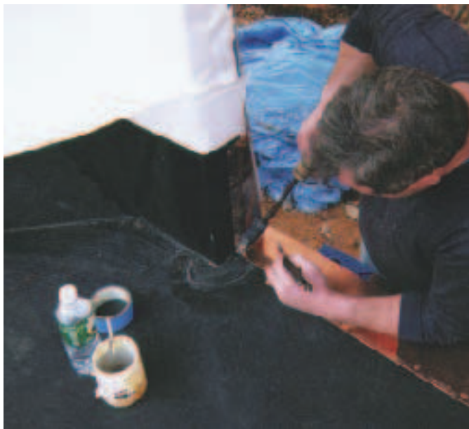
Figure 5. A soldered copper drip pan, nailed on top of the membrane, is sealed under a self-sticking rubber flashing strip. A pliable self-sticking uncured rubber patch seals the junction of the outside wall corner and deck (left). The drip pan directs runoff into a copper gutter (right).
